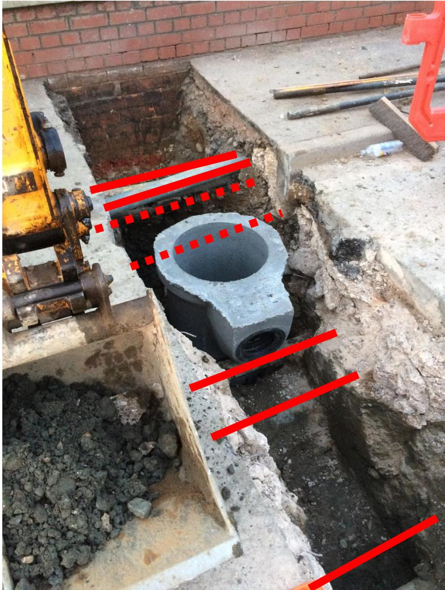
The excavations have been backfilled using both foamed concrete and a granular material depending on whether there was room for compaction of the material. Permanent reinstatement of the carriageways and footways has been carried out using a polymer modified mastic asphalt highway reinstatement system. All drainage works in Phase 1, which are outside of the newly resurfaced area, are programmed for completion on Sunday 12<sup>th</sup> August 2018.
